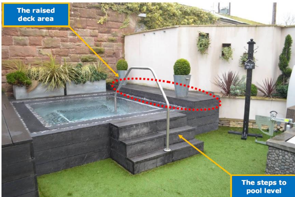
Photograph 2 The incident locus, with the raised deck area and the steps to the pool level indicated.
