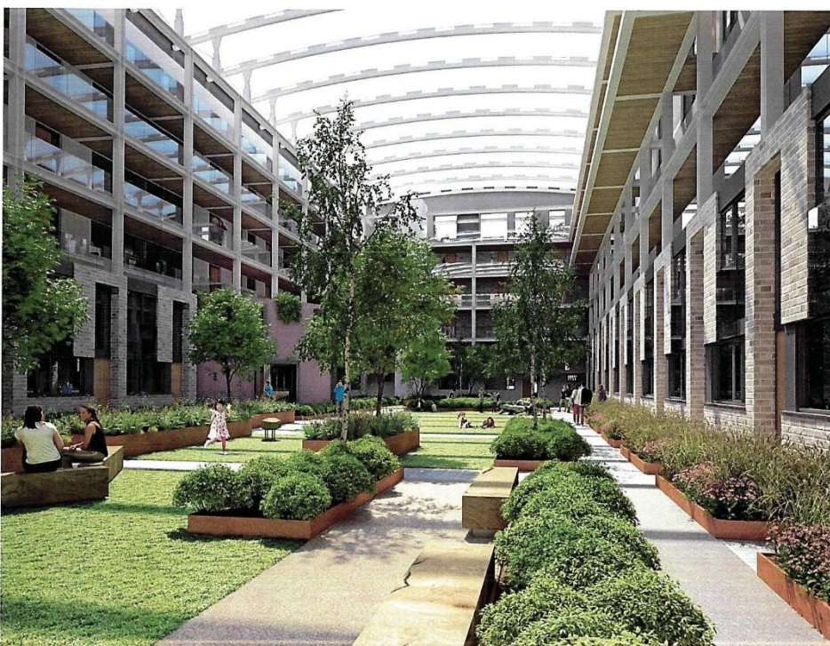
Figure 2 – Internal Courtyard – general view facing Southeast.
